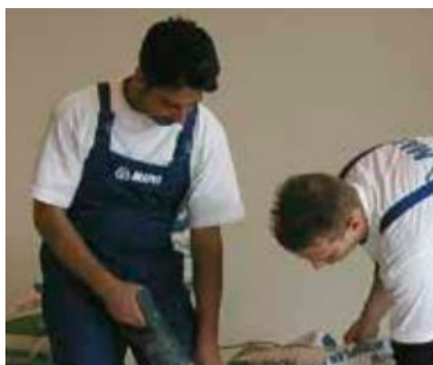
Mixing Ultraplan Eco - Mirabello kindergarten - Cantù (Como) - Italy
