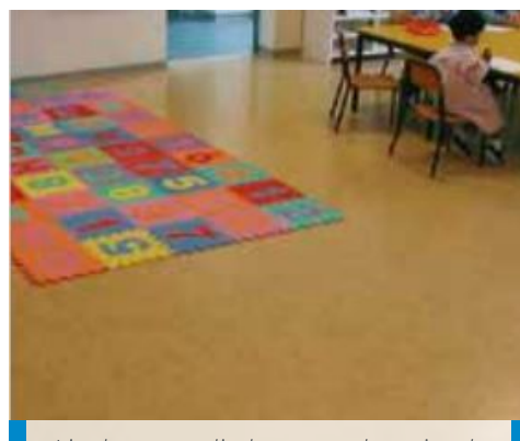
Linoleum applied on screed previously levelled with Ultraplan Eco - Mirabello kindergarten - Cantù (Como) - Italy
