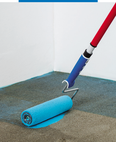
First coat application of Mapeproof Primer
