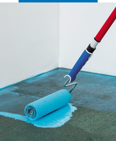
Second coat application of Mapeproof Primer
