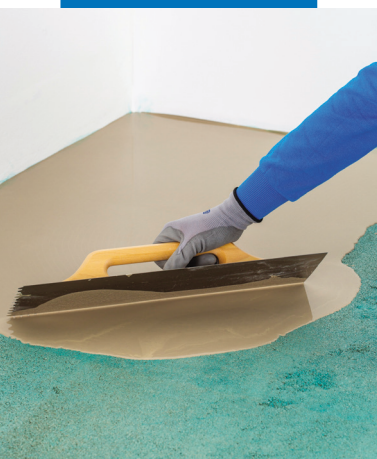
Self-levelling compound application on Mapeproof Primer
