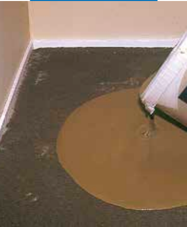
Applying the Novoplan 21 paste on the substrate
