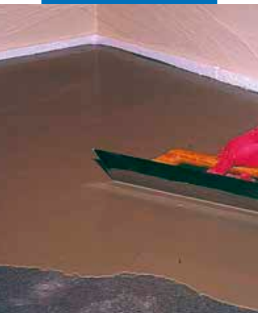
Applying Novoplan 21 with a metal trowel on a cementitious screed primed with Primer G
