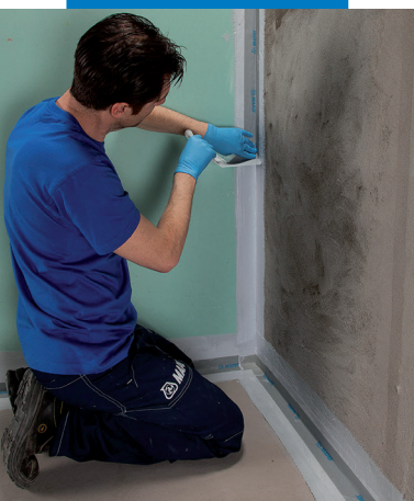
Application of Mapeband PE 120 using Mapegum WPS
