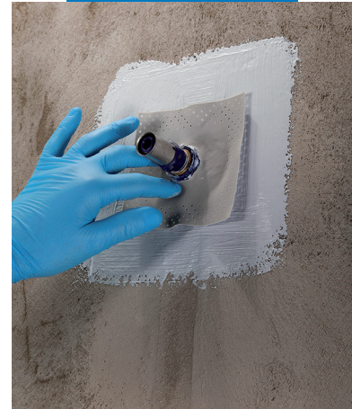
Application of a Mapeband PE 120 seal for through holes using Mapegum WPS
