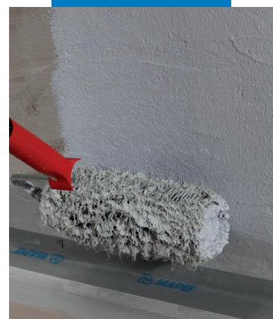
Application of Mapegum WPS with a roller
