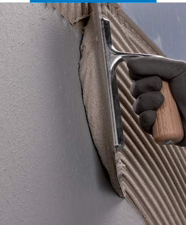
Installing floor covering using Ultramastic III
