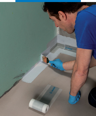
Application of Mapeband PE 120 using Mapegum WPS
