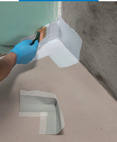
Application of a 90° Mapeband PE 120 corner piece using Mapegum WPS
