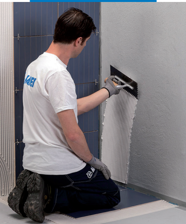
Installing wall covering using Keraflex Maxi S1
