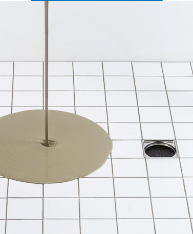
Application of Planex HR on existing ceramic tiles in damp surroundings
