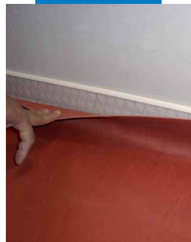
Forming a fillet shell using Mapecoat
