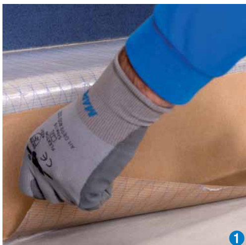
Positioning Mapecoat on the riser of a step
