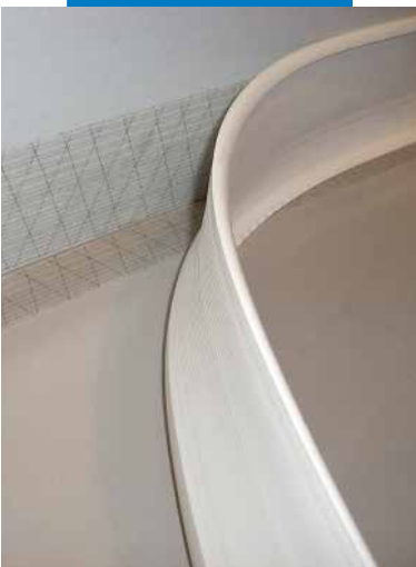
Application of a plastic-coated PVC skirting board using Mapecontact
