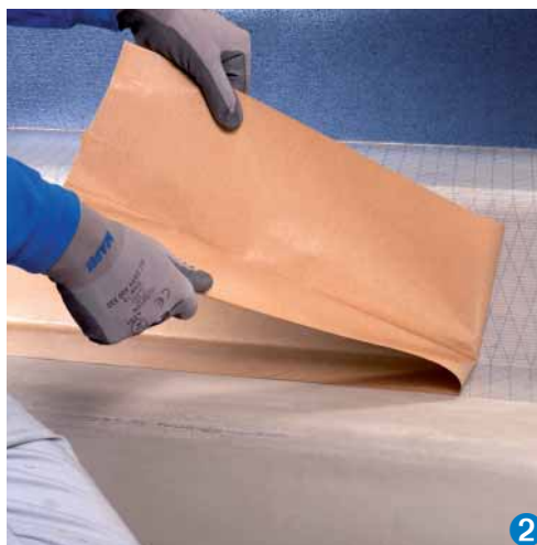
Removal of the protective coating
