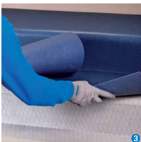
Application of PVC on steps using Mapecoat
