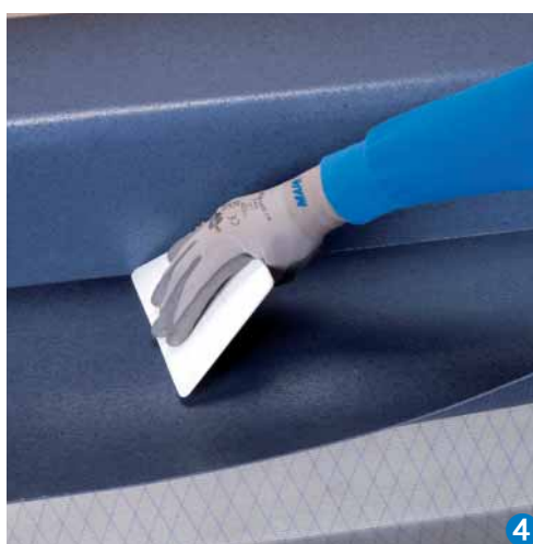
Massaging the PVC after applying Mapecoat
