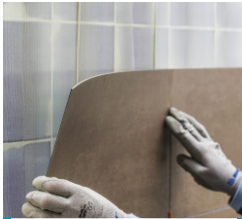
Installation of LVT on a wall
