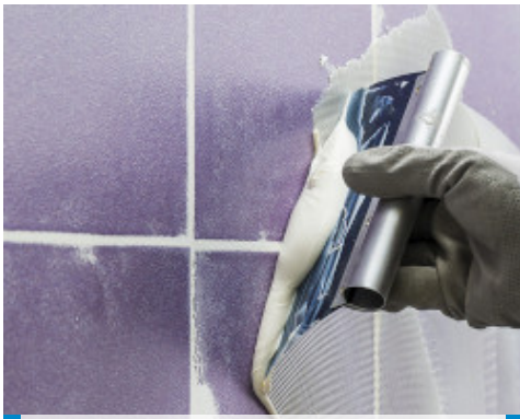
Spreading Ultrabond Eco MS 4 LVT Wall with a notched trowel on a non-absorbent substrate
